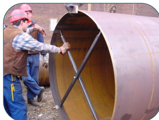
Fig 1: Cross-Bracing in pipe
